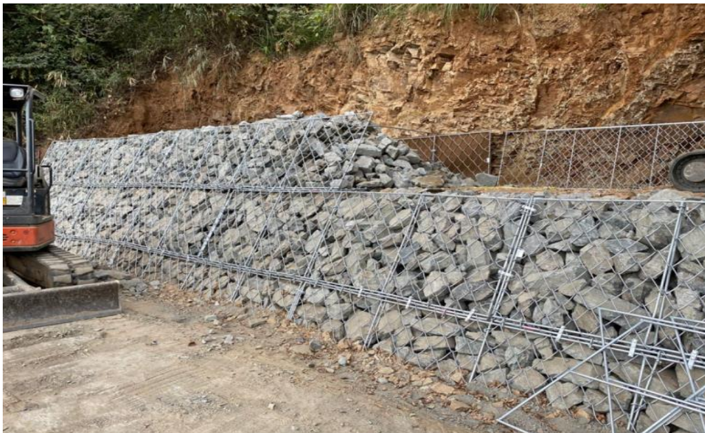
Figure 6.11 Gabion Check Dam (Source: Pinterest Gabion Check Dam)
